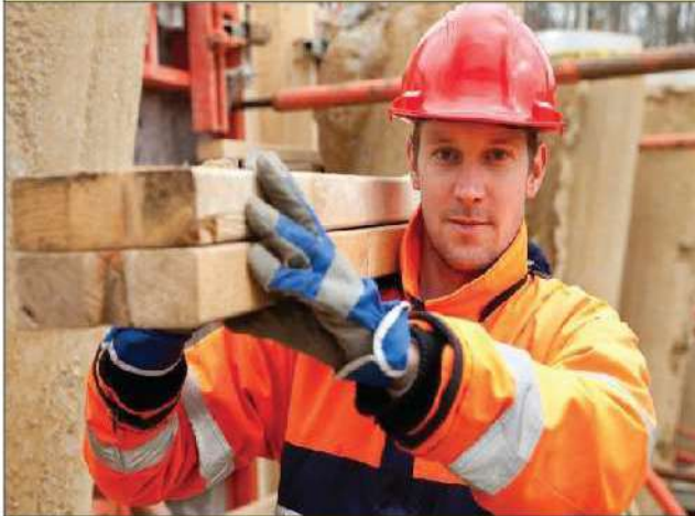
Our workers are working in construction sector
